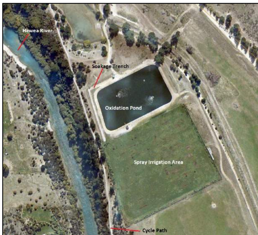
Figure 1.2: Overview of Wastewater Treatment Plant
