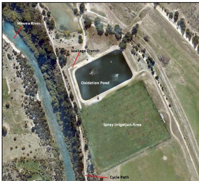
Figure 1.2: Overview of Wastewater Treatment Plant
