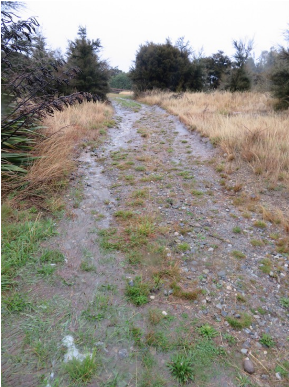
Figure 4.3: Water eroding 4wd access track to Kirsty's beach (26/3/19)
